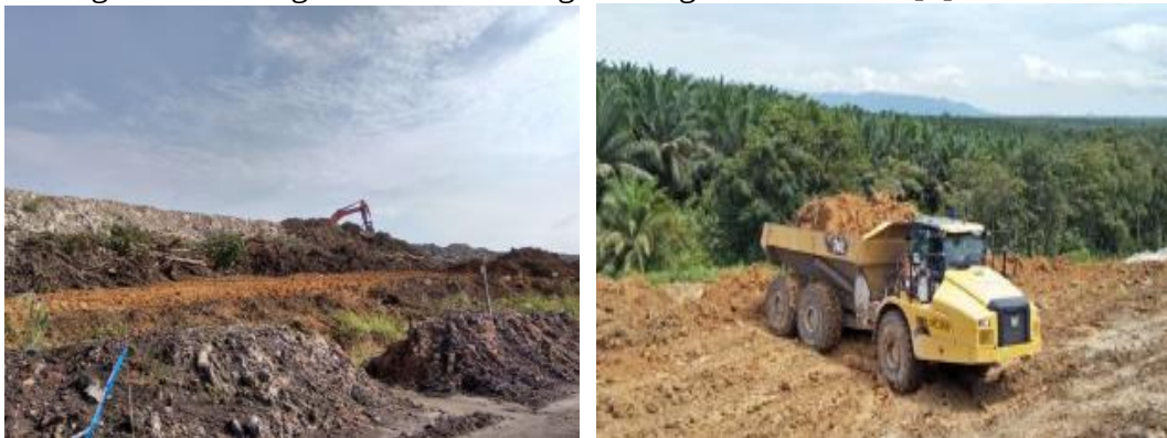
Gambar 2. Tahapan Overburder Removal
